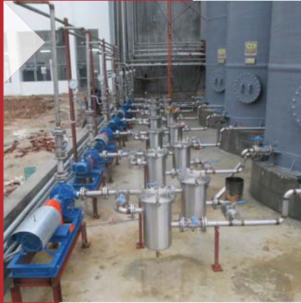
"Gear Pump" CP Vietnam Corporation - BINH DINH Feed Mill Branch, Vietnam
