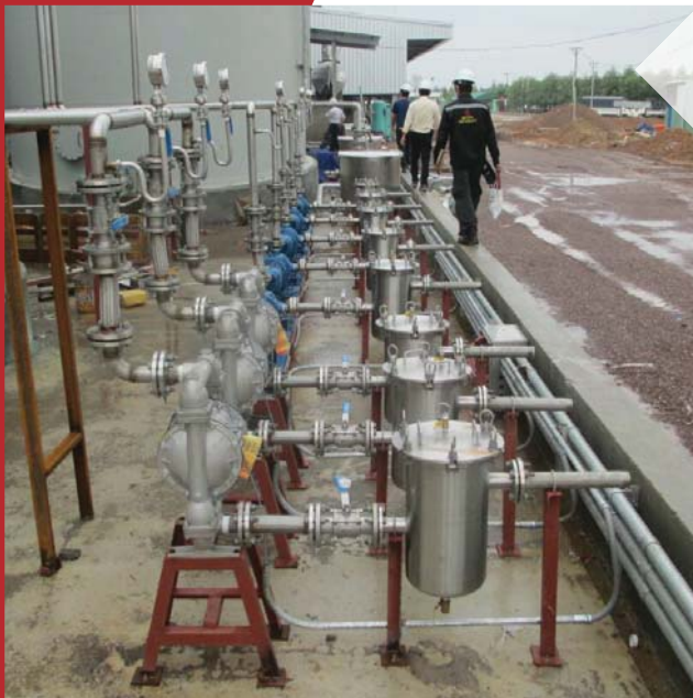
"Air Operated Double Diaphragm Pump" CP Vietnam Corporation - BINH DINH Feed Mill Branch, Vietnam
