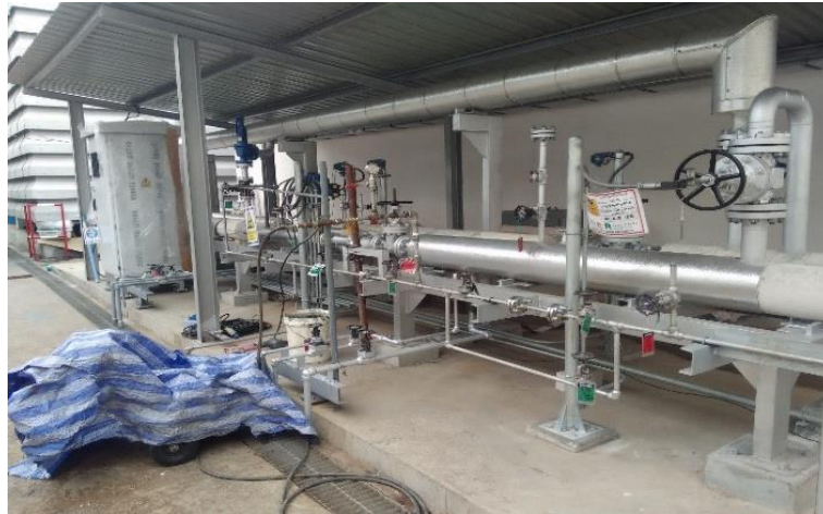
Metering and Letdown system of Nava Nakorn Electricity Generating Company Limited (NNEG)
