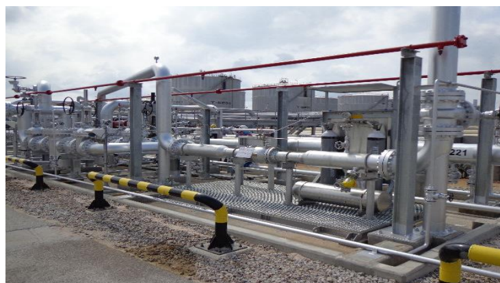
Emergency Pressure Relief System for Oil Pipeline System of PTT Global Chemical Public Company Limited
