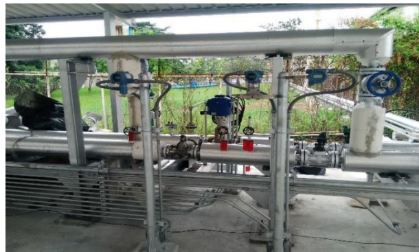
Metering and Letdown system of Bangpoo Cogeneration of Eternal Energy Public Company Limited
