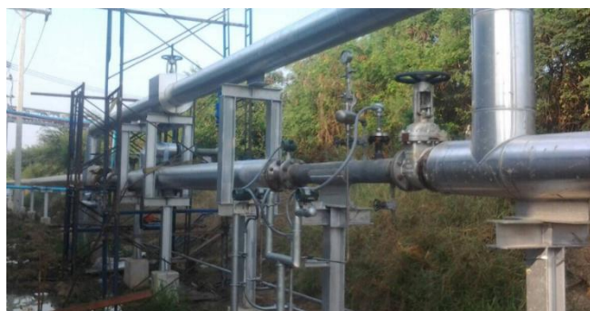
Metering and Letdown system) Ratchaburi World Cogeneration Company Limited
