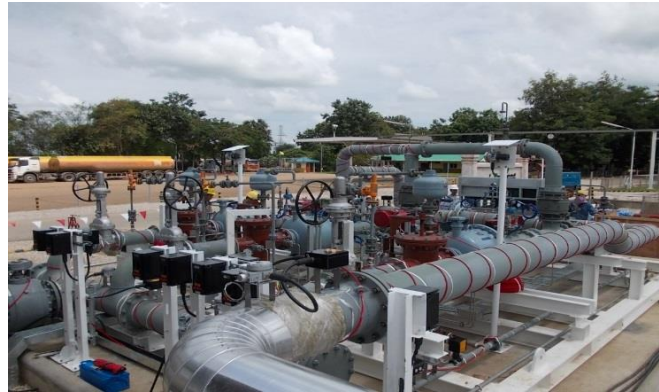
Crude Oil Metering System and Electrical Heat Tracing Cable of PTT Exploration and Production Public Company Limited
