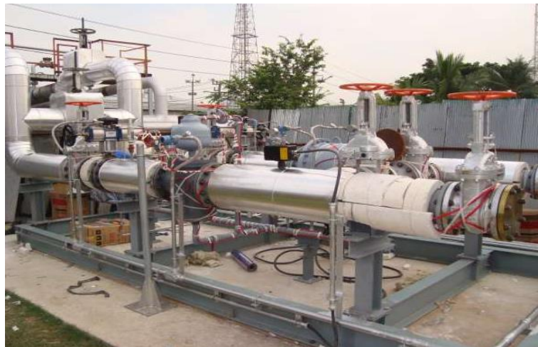
Metering System for Heating Oil / Gasoline 91/95 and Electrical Heat Tracing Cable of Bangchak Corporation Public Company Limited
